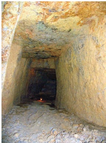
Fig. 6. Roșia Montană: an ancient drift of typical trapezoidal section in the Cărnic massif.
