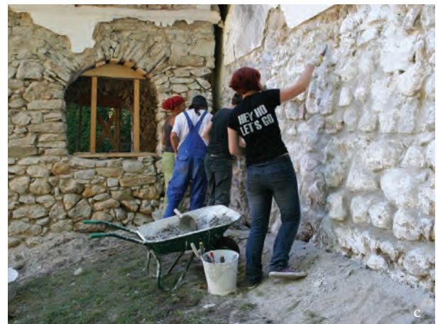
Fig. 4. Roșia Montană , Alba: a. Open-air theory and practice lecture in the Unitarian parish yard (2009); b. Practical conservation work in the Unitarian parish house - cleaning masonry joints (2010); c. Practical conservation work at the Unitarian church - repointing (2011).
