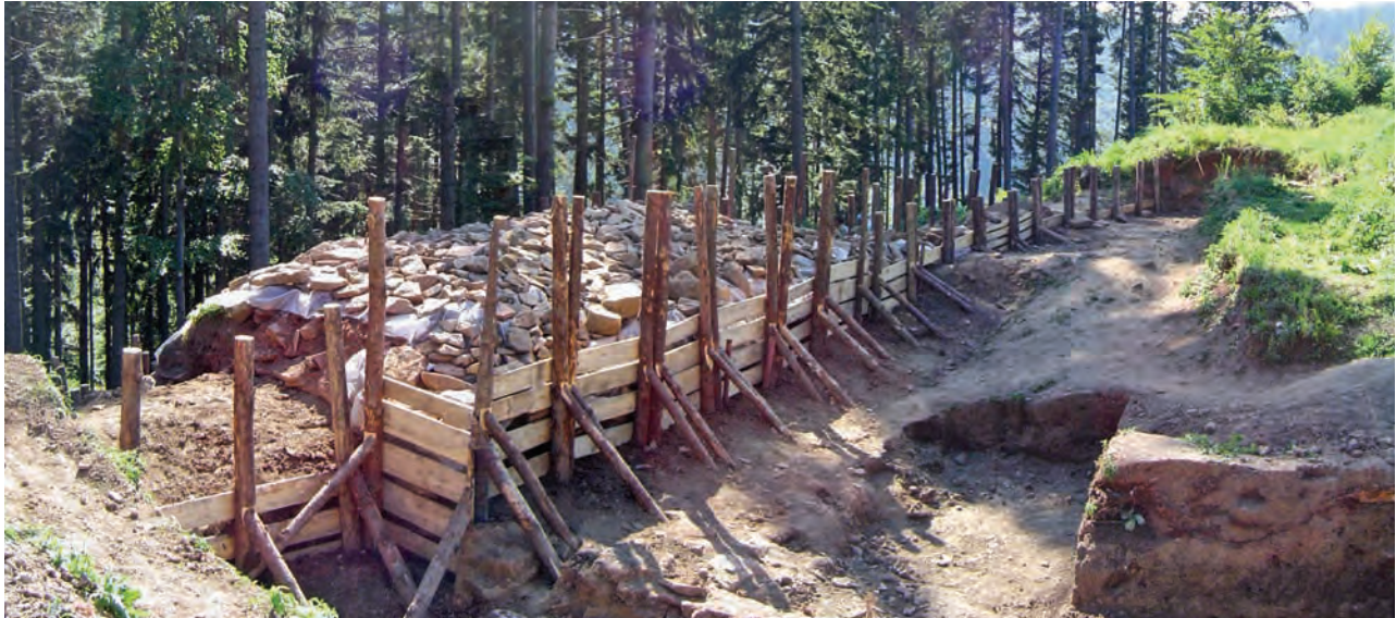
Fig. 1. Cetatea Zânelor, Covasna: emergency protection of the fortification wall of terrace 2 (2006).
