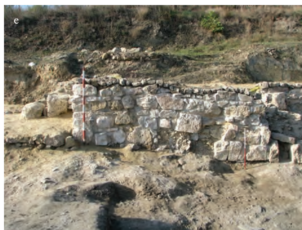
Fig. 6. Nufăru , Tulcea: the landing area facing the Danube. a. The situation prior to the conservation works (2010); b. The archaeological area at the end of the intervention (2012); c, d. Consolidation of masonry by cleaning the joints and re-filling with mortar; e. the main tract of wall after completion of works (photo: M. Vasile).
