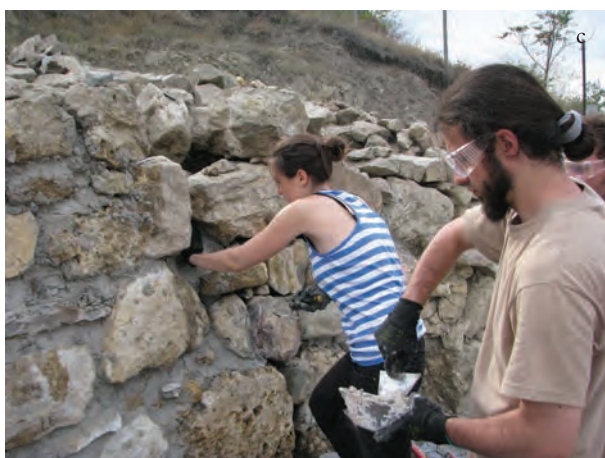
Fig. 6. Nufăru , Tulcea: the landing area facing the Danube. a. The situation prior to the conservation works (2010); b. The archaeological area at the end of the intervention (2012); c, d. Consolidation of masonry by cleaning the joints and re-filling with mortar; e. the main tract of wall after completion of works (photo: M. Vasile).
