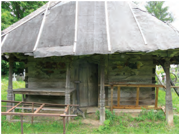
Fig. 4. View toward the porch of the church.
