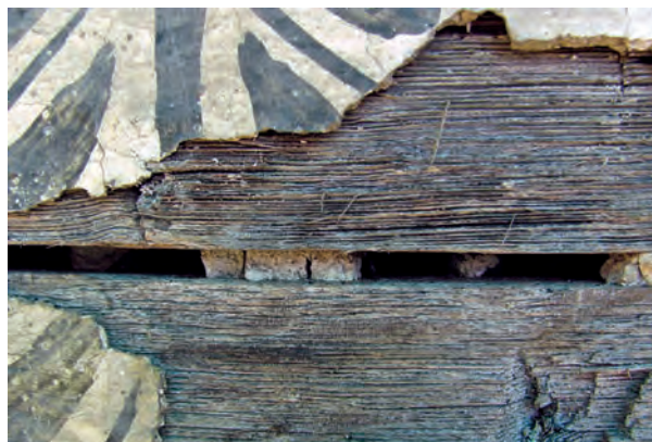
Fig. 21. Spaces between logs were sealed with the same type of mortar used for the support of the al fresco painting.
