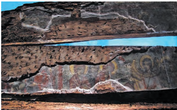
Fig. 27. Degradation of wood exposed for a long time to infiltration humidity, and displacements of vault planks resulted in wide losses of the fresco painting.
