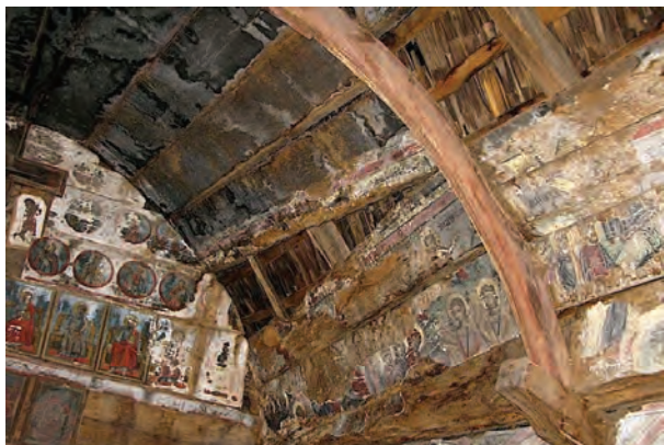
Fig. 24. The south-eastern area of the naos vault with complex degradations of the wood, fresco painting and al secco painting of iconostasis.
