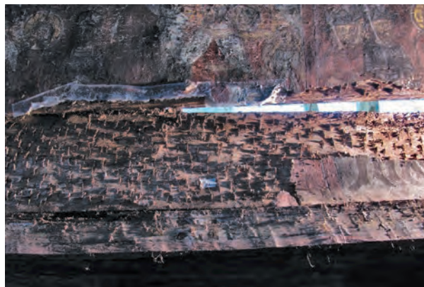
Fig. 20. Adze or hatchet strikes cut into the oak logs to provide a hooking surface for the support-plaster of the al fresco painting.
