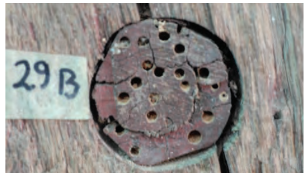
Fig. 36. Flight holes on the wood in the naos.
