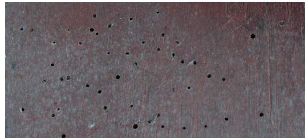
Fig. 35. Flight holes on the wood of the iconostasis.
