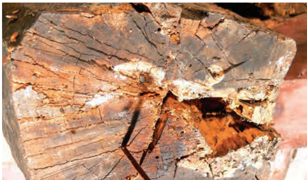
Fig. 33. Extended mycelium of basidiomycetes and flight holes.
