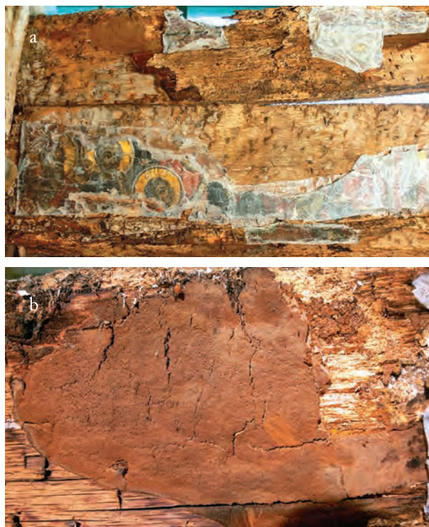
Fig. 37 a, b. Fructification bodies and mycelium of Antrodia sinuosa (photo V. Albu).
