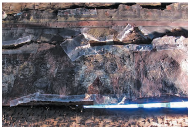
Fig. 25. Raking light highlights both the dislocations of the vault planks and the detachments and the lacunae of the fresco painting.
