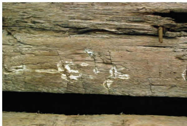
Fig. 31. Basidiomycetes mycelium and flight holes (photo V. Albu).
