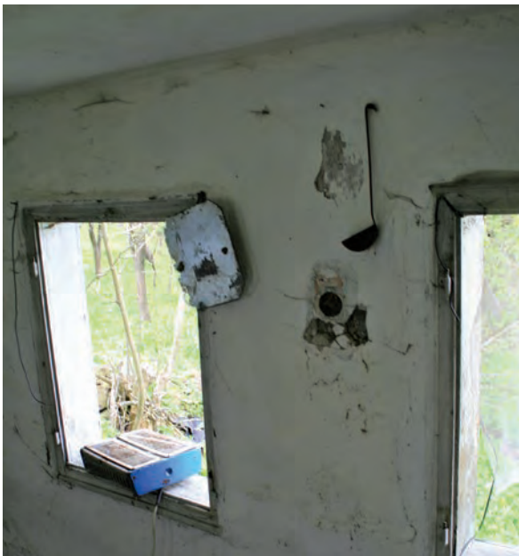
Fig. 15. Roşia Montană, May 2008: House 519; the first room (photo: Radu-Alexandru Dragoman).
