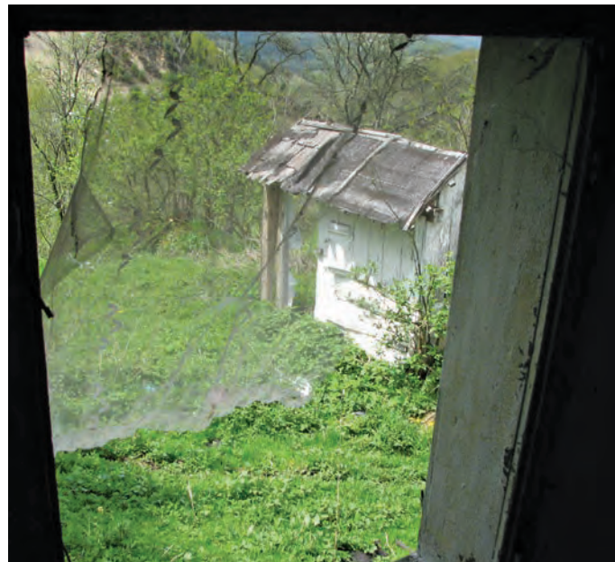
Fig. 16. Roşia Montană, May 2008: House 519; outlook through one of the windows of the first room (photo: Tiberiu Vasilescu).
