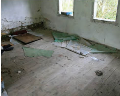
Fig. 12. Roşia Montană, May 2008: House 519; the first room (photo: Radu-Alexandru Dragoman).
