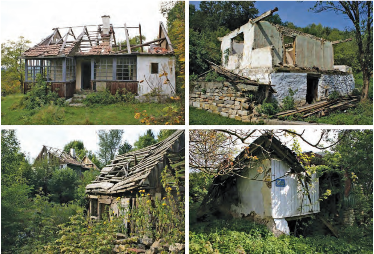
Fig. 20 . Historic houses demolished or abandoned to self-destruction in the Sosași neighbourhood, adjacent to the historic centre, in the proximity of the Market Square and elsewhere within the historic town. The blue plate on the house in the lower right corner reads: Property of the Roșia Montană Gold Corporation.
