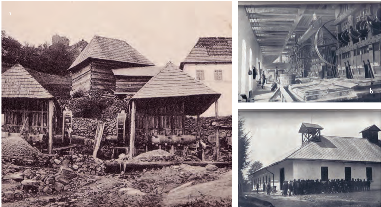
Fig. 7. Processing structures and plant: a. Historic stamping mills; b. The processing plant at Gura Roșiei built in 1851-1852; c. 19 th c. roll-call and shaft house at the state mine (a. historic photograph, beginning of 20 th cent.; b, c. Zotinca 1928).
