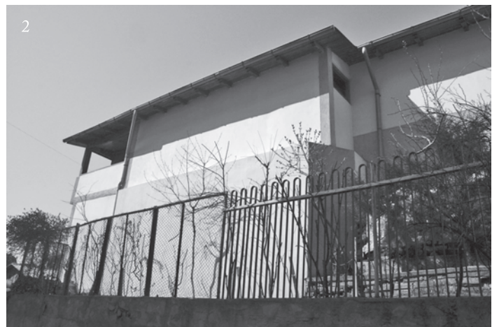
Fig. 15. Mangalia blockhouse incorporated in a residence (April 2012).
