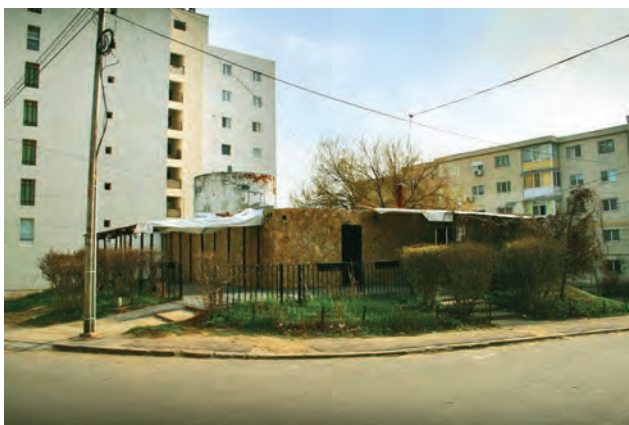
Fig. 12. Blockhouse from Constanța transformed into a bar (April 2012).
