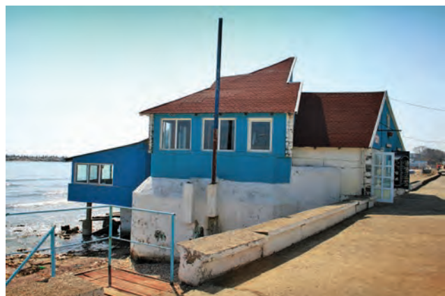
Fig. 13. Blockhouse from Mangalia transformed into the restaurant Puius Cazemată (April 2012).
