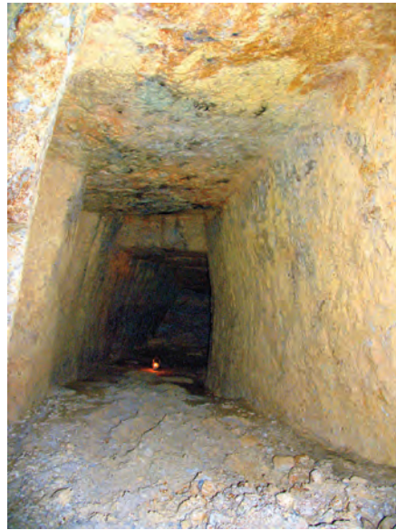
Fig. 6. Roşia Montană: an ancient drift of typical trapezoidal section in the Cărnic massif.
