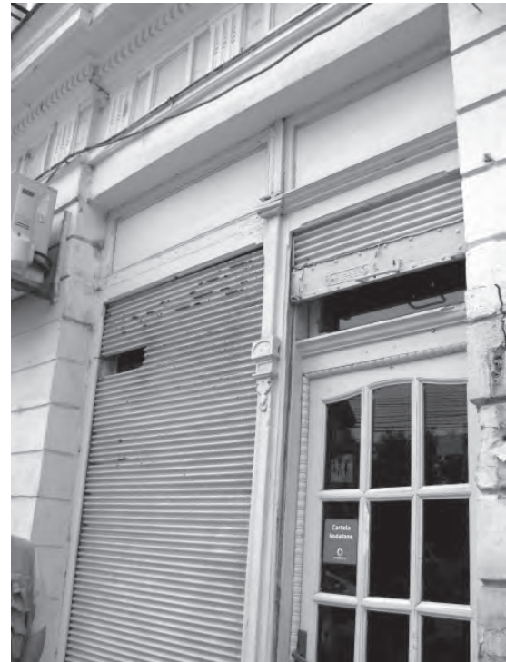
Fig. 6. Rollingshutters J. Haug, Colţei Street No. 3.
