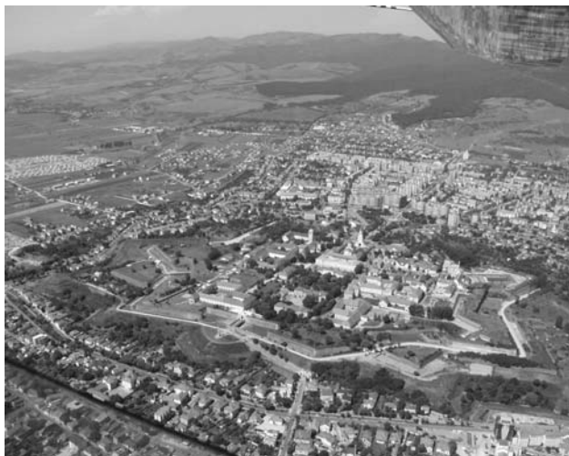
Fig. 12. Alba Iulia: buildings sprawling on the Romans' Plateau and in the glacis of the Vauban fortress (aerial photo by I. Bogdan Cataniciu, June 2009).
