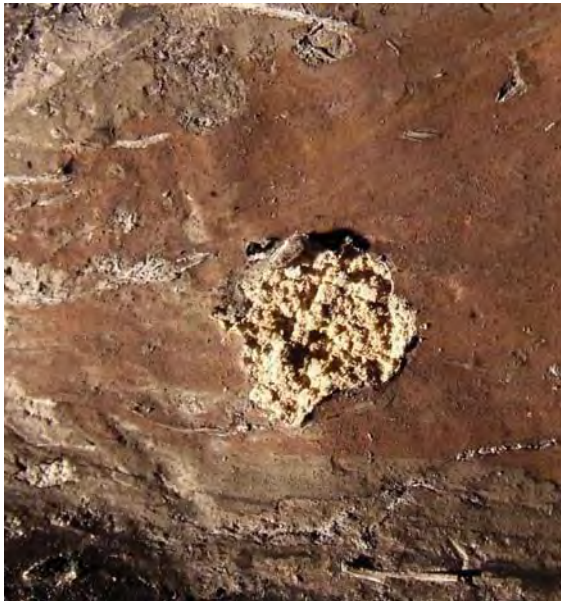
Fig. 4 a. Incipient signs of cohesion loss of the pictorial strata and of the support, point shape. The porch of the Humor Church.
