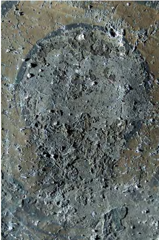
Fig. 8 a, b, c, d. Different morphologies of gaps as result of the adherence and cohesion loss of pictorial stratum in the porch of Doamnei Church (a, b, c) and in the porch of Humor Monastery, where a selective disappearance of the tone of the colour stratum can be noticed.
