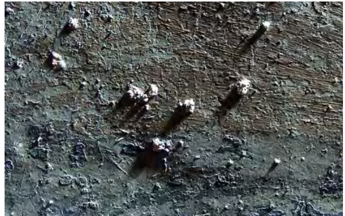
b. Point shape craters which appeared due to an older process of defoliation of the pictorial stratum. The porch of Doamnei Church.
