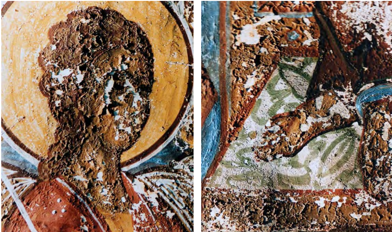
Fig. 7 c, d. Different morphologies of defoliation in the porch of Humor Monastery Church.
