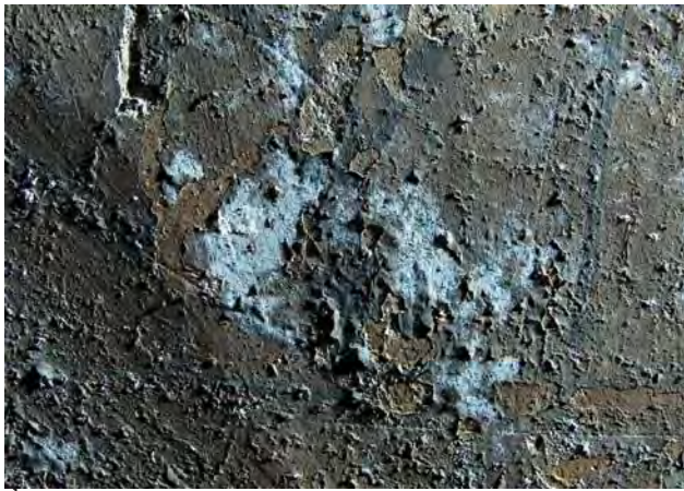
Fig. 6 b, c, d. Macro photos illustrating the process of the appearance of efflorescent crusts on the surface of pictorial stratum. The porch of Doamnei Church.
