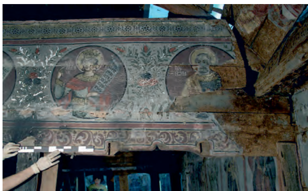
Fig. 1. Beam no. 2 shows the characteristic morphology of the biodeterioration process.
