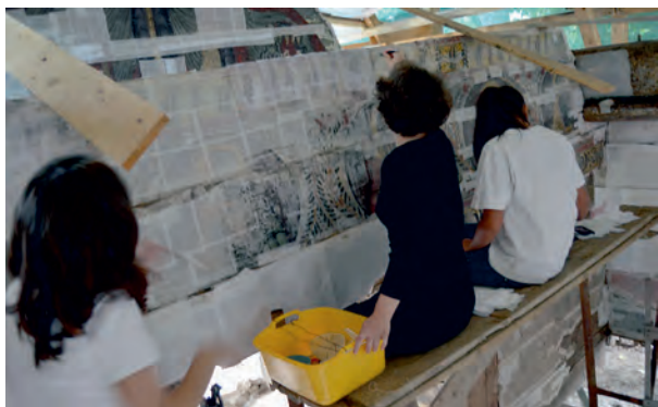
Fig. 2. Securing the pictorial layer before removing beam no. 2.
