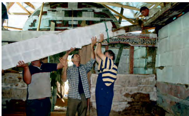
Fig. 3. Dismantling of beam no. 2.
